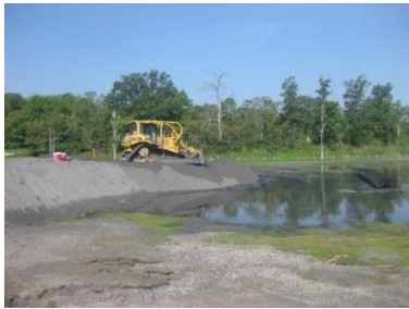
Step 1: Start of Access Road Geogrid and Bottom Ash
